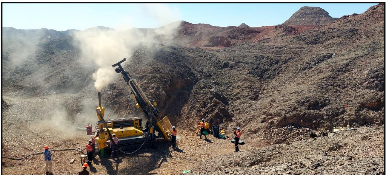
Figure 2: Capital Limited's Explorac 100 RC rig collaring off the first hole HAP-101
