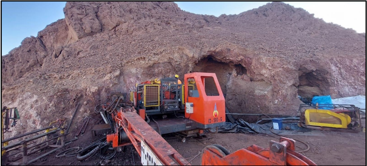
Figure 2: Horizontal drilling on hole ROD-066, under the South Ridge summit line
