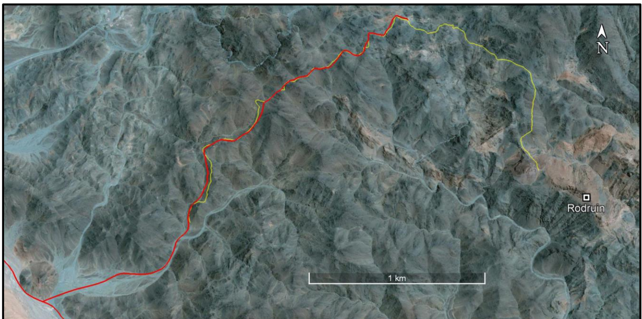
Figure 4: Rodruin access road, as of April 13, 2018 (red: actual position of road; yellow: planned route of road)
